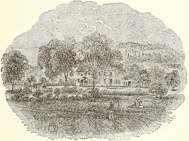
MANSION HOUSE, NEW IPSWICH. Built by Col. Reuben Kidder, about 1754.
